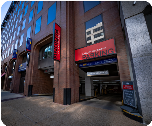
Parking garage entrance from 20th Street
