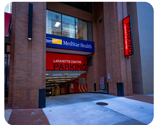
Lafayette Centre 21st Street garage entrance
