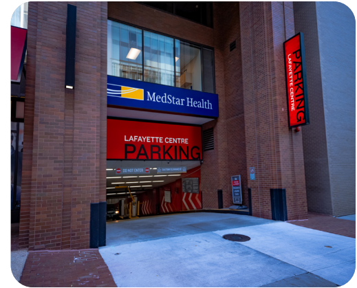
Lafayette Centre 21st Street garage entrance
